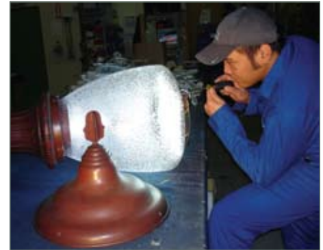
Raymon Salamanca, Designer/technician, installs a test LED light engine in a popular "acorn fixture"
