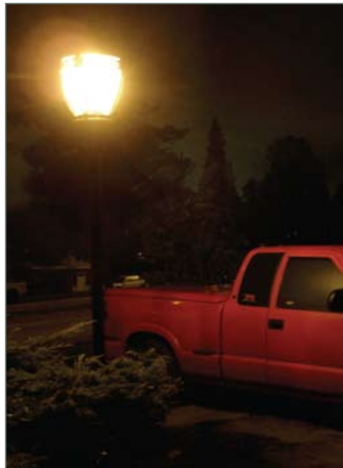
75 Watt high pressure sodium before conversion. Total wattage: 87 watts
