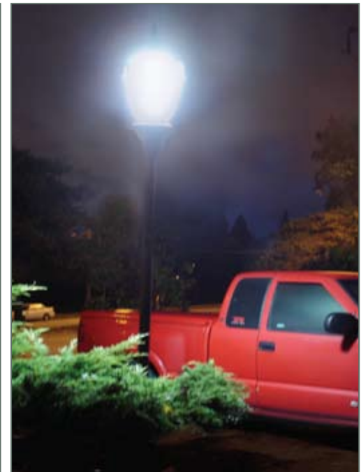
32 LED fixture after conversion, Total wattage: 43 watts
