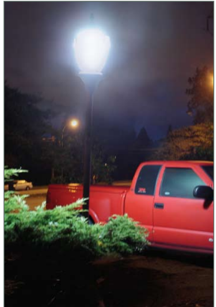
40 Watt LED's after conversion. Total wattage: 44
