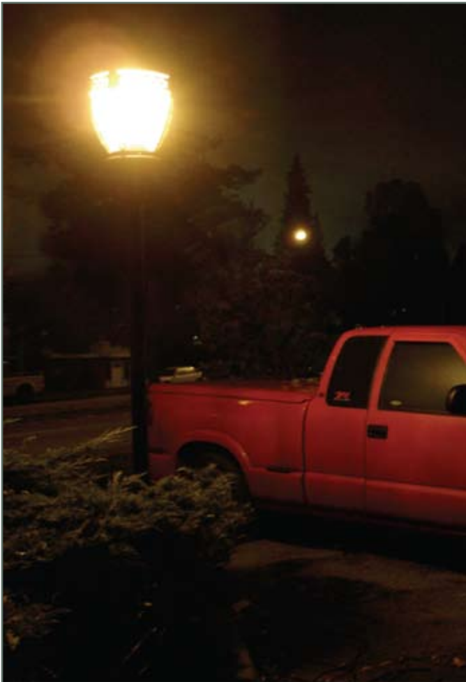
70 Watt high pressure sodium before conversion. Total wattage: 81
